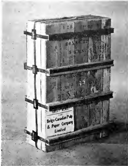
8.—Small bales ready for shipment. These bales are made for transportation on mule or horseback.
